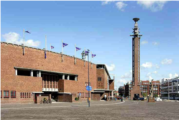
Figure 1 Olympic Stadion Amsterdam (1928)
